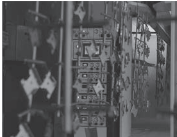
Robotics Paint Facility
